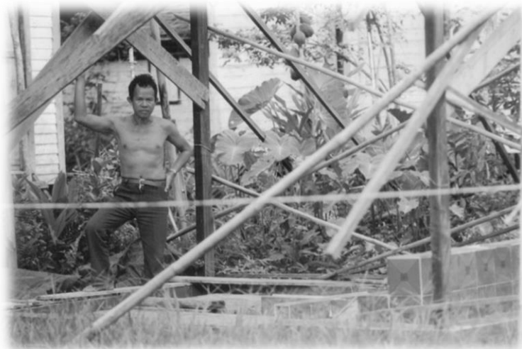
Pid'jer's Grave - with roof under construction
